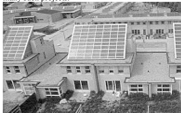
PV Roof Installations on Luxury Owner-occupied Houses in Amersfoort (photograph courtesy of REMU)
