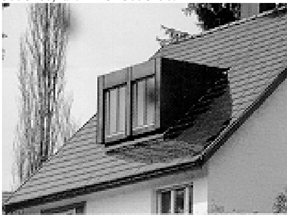
Residential House in Basel, Switzerland (photograph courtesy of Atlantis Solar Systems Ltd)
